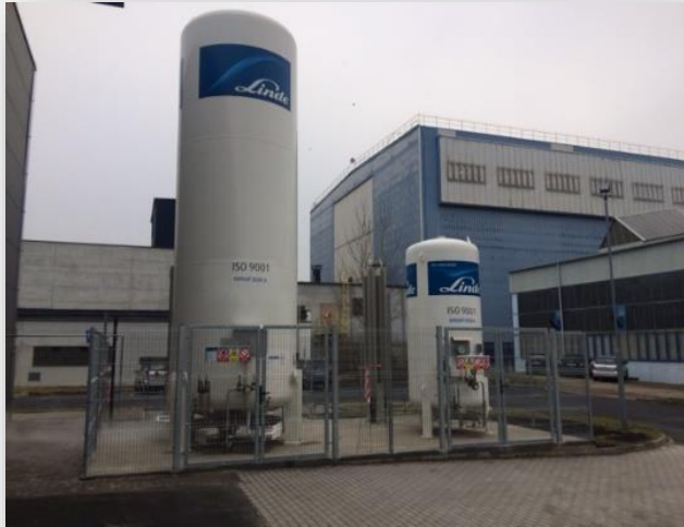
High capacity gas storage (Nitrogen, Oxy) in place from December 13th 2019
